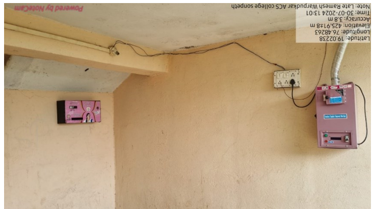
For girls near washroom equipped with sanitary napkin vending and destroying machine
